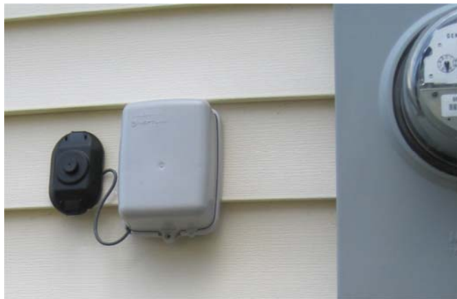
Left: The TRF-W Provides Water Utilities With The Flexibility Of Reading Meters Using Either An AMI Radio Endpoint or a Touch-Read Pad.
